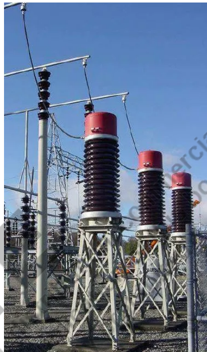
Fig. 5.11: Potential Transformer (a) Symbol, (b) PTs in substation
